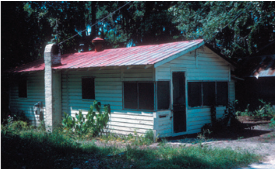
Figure 10: The second house that Murrill built
